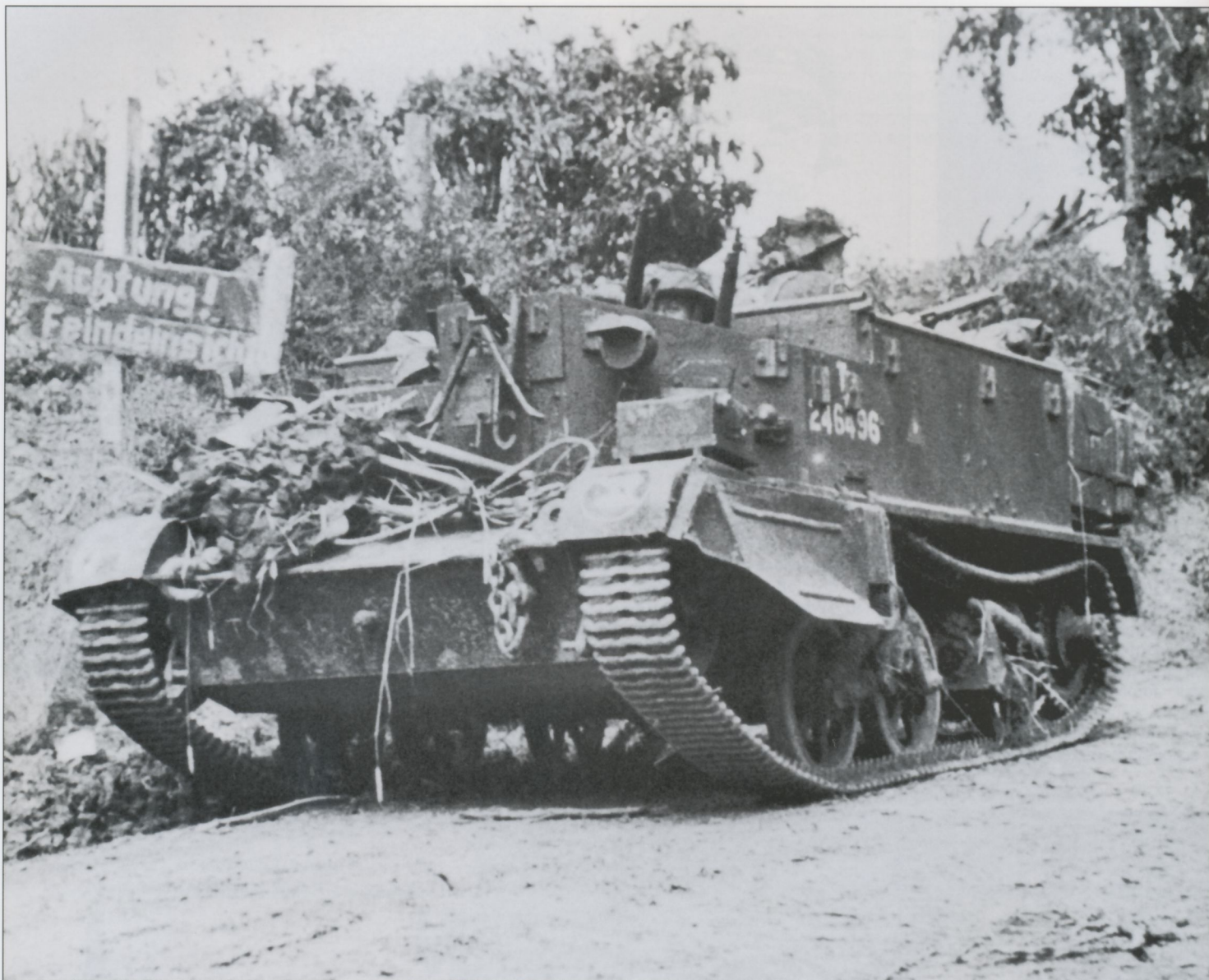
A British Universal Carrier driving in the Cheux area in late June 1944. Note the captured MG42 projecting from the driver's compartment. The formation badge of the 49th (West Riding) Infantry Division, a white polar bear standing on an ice floe, is painted on the left trackguard of the carrier. The Arm of Service number, '64' is painted in white on a black square on the right trackguard. The sign in the background, 'Achtung! Feindeinsicht' warns the enemy can observe your movements.
